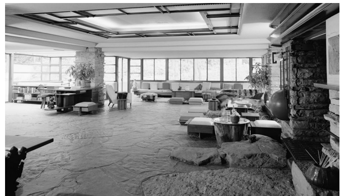
03 Fallingwater. The living room opens towards the woods. Jack E. Boucher, 1985 · Library of Congress, HABS 1-48
